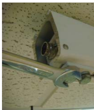
1.6 Loosen end stop bolts
